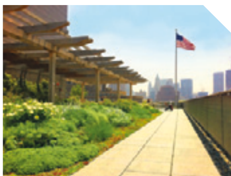
View of the “green roof” on the office building where Edelman New York operates.
